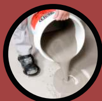
Flooring Levelling
